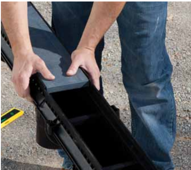
3. Ensure that channels are securely connected and correctly aligned
