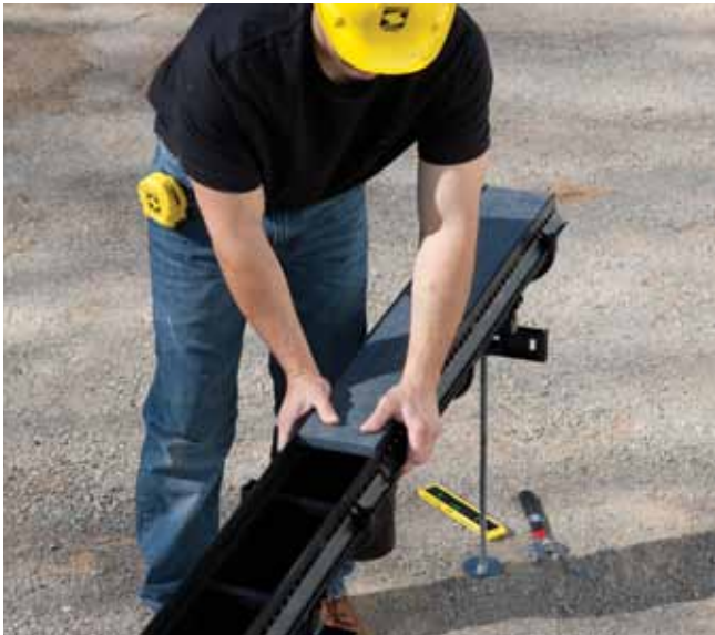
3. Ensure that channels are securely connected and properly seated in the Rante Arrow.
