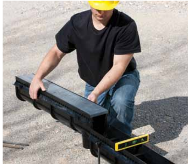
2. Slide channels together.
