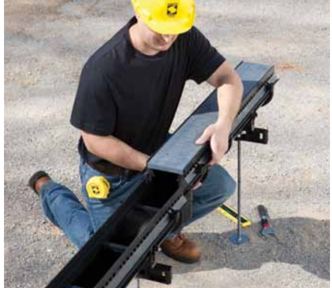
2. Slide channels together.
