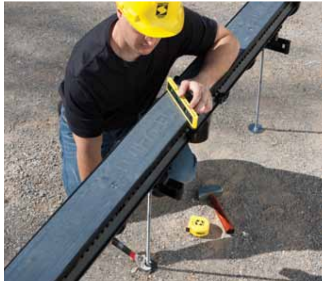
4. Check for level to ensure that channels are installed properly.
